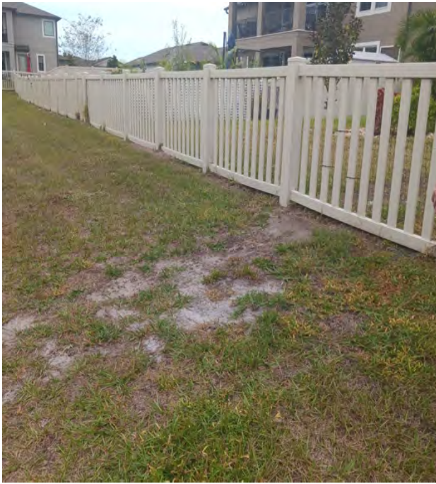
18005 Cortes Creek pop-up drainage
